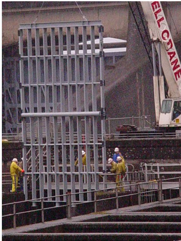
Appendix 2. Sea lion exclusion device (SLED) at Bonneville Dam fishway entrance (A) and installed (B), floating orifice gate (FOG) (C), and sea lion incursion barriers on top of FOGs (D).
